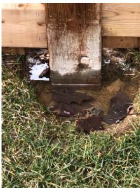
b) Water will sit on top of the concrete, below grade and over time rot the post. (as you can see in the photo)
